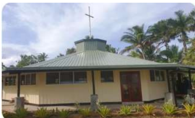
2020 facelift with new colourbond roofing, new windows, and posts
