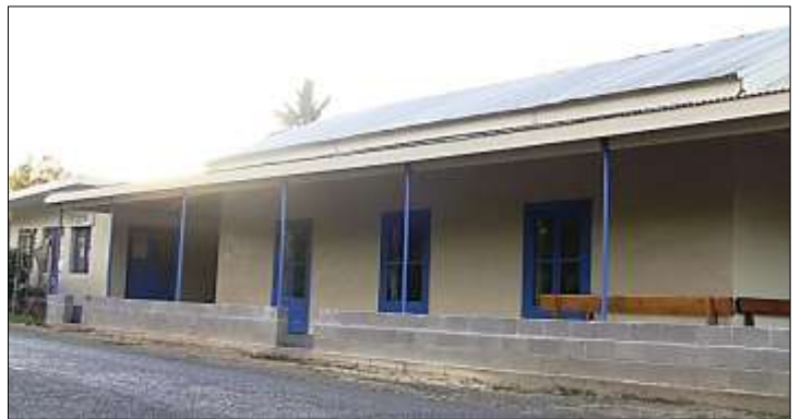
"Ebenezera" & the Avatiu Clinic under renovation.
